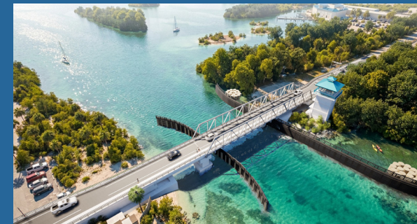
Single-Lane Swing Span Bridge with One Sidewalk
