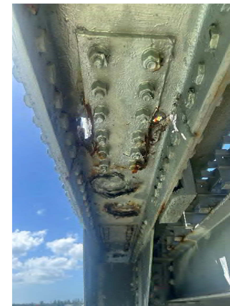
Photographs representative of existing conditions of the swing bridge's main lower truss members
