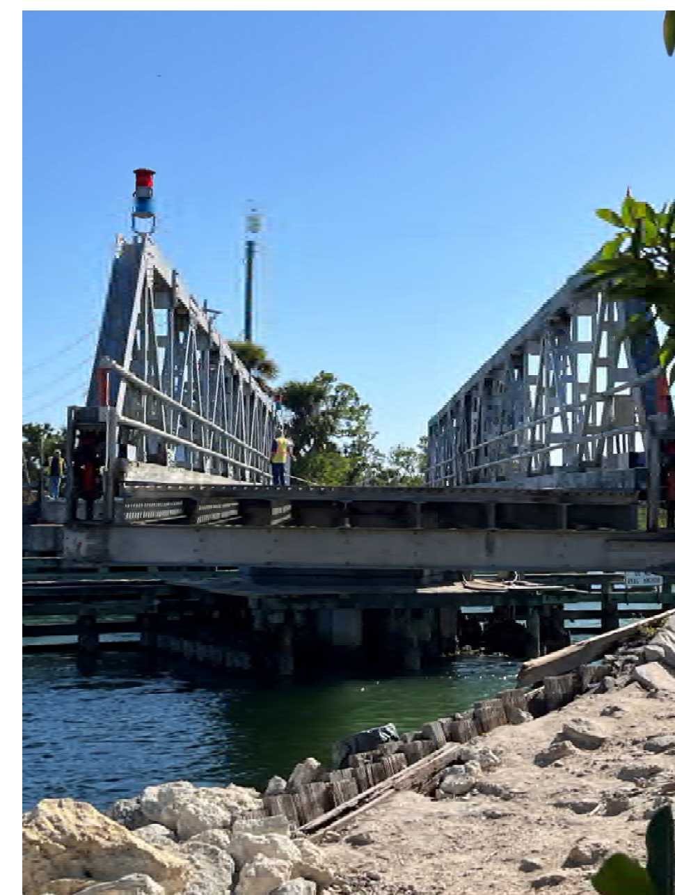
Failing Timber Retaining Wall
