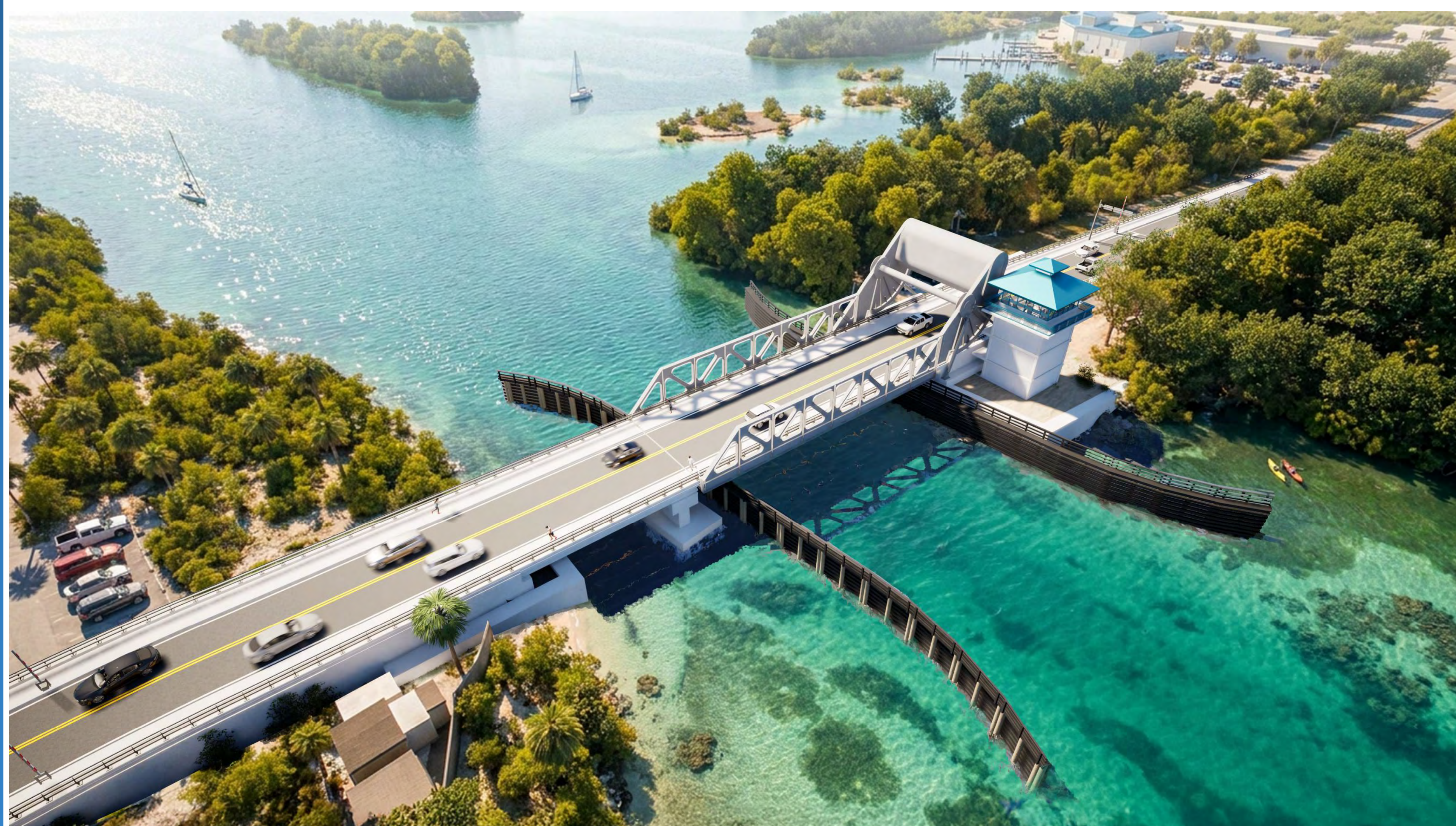
TWO-LANE BASCULE BRIDGE WITH TWO SIDEWALKS
