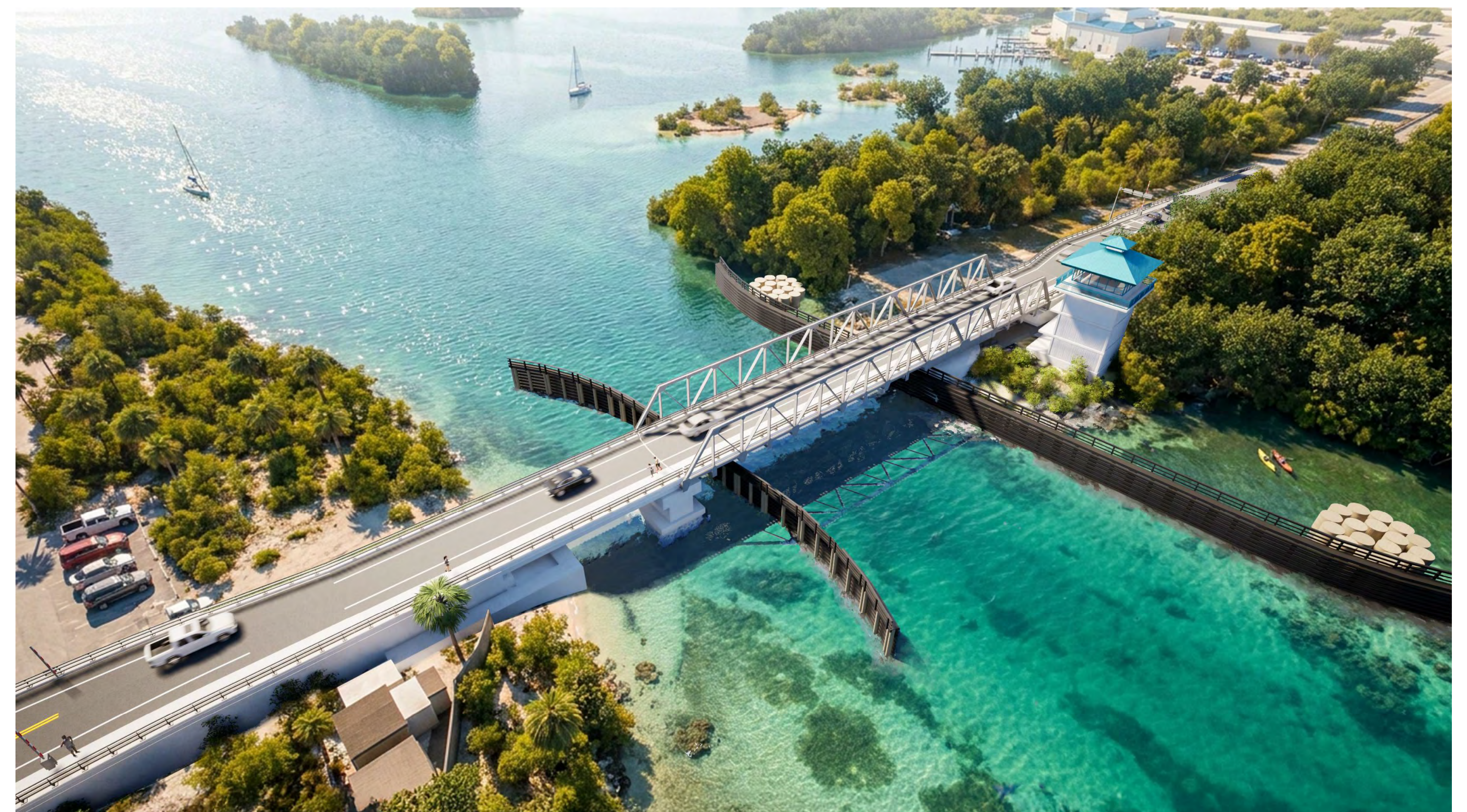
SINGLE-LANE SWING BRIDGE WITH ONE SIDEWALK
