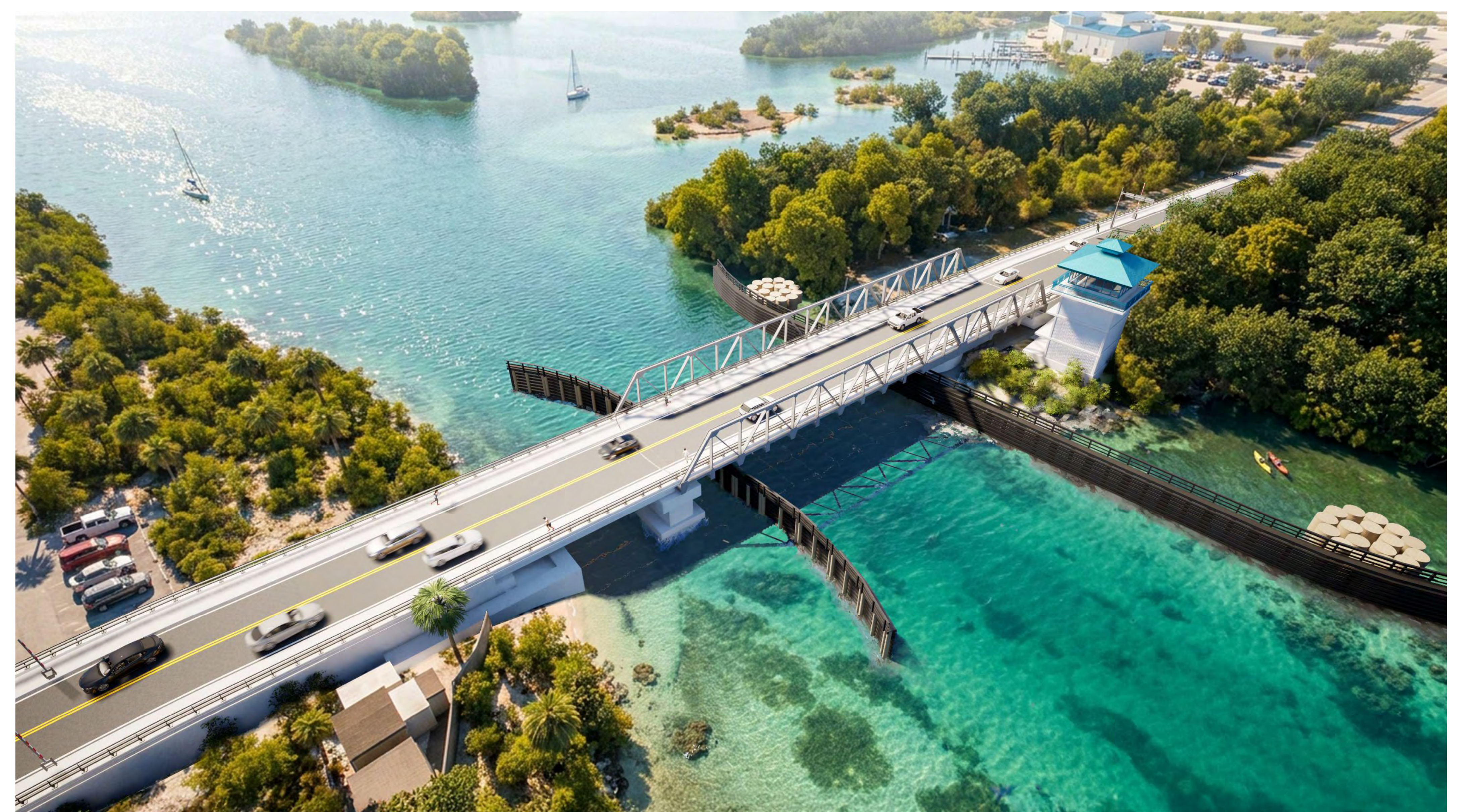
TWO-LANE SWING BRIDGE WITH TWO SIDEWALKS
